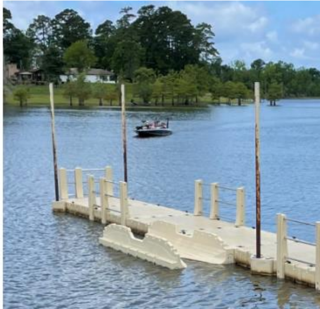
Kayak launch and handrail installed within the Region at a different lake.
