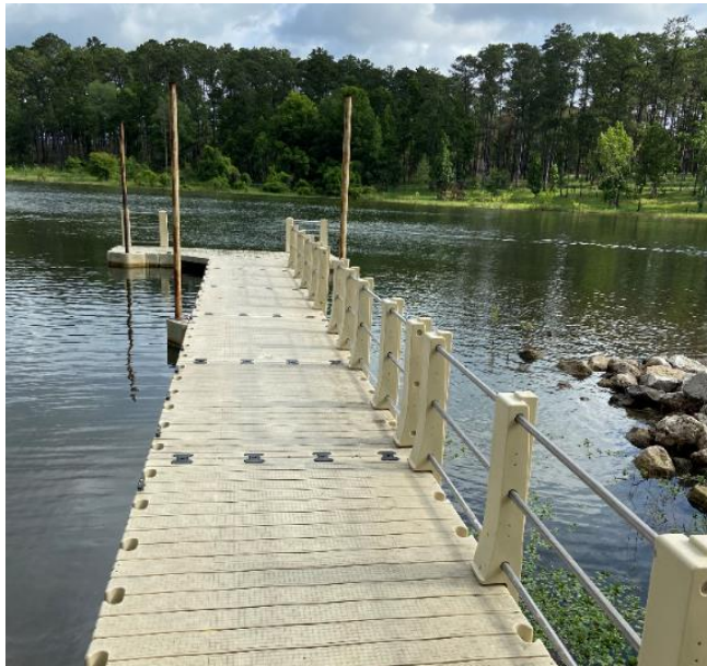
Handrail installed within the Region at a different lake.
